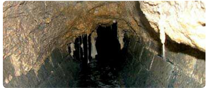
Fat and grease that is not dealt with correctly could have this effect on our sewers.
